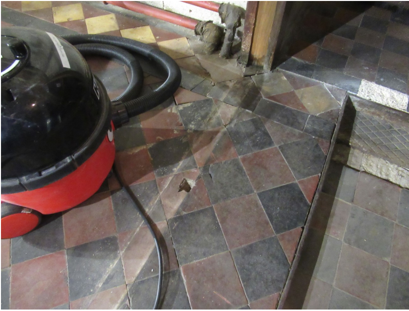
A hole in the floor where a bolt from the South door would have slotted in to before the 'box' was built.
