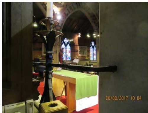
Fig 7 Wrought iron rail – horizontal bar and scroll at north end
