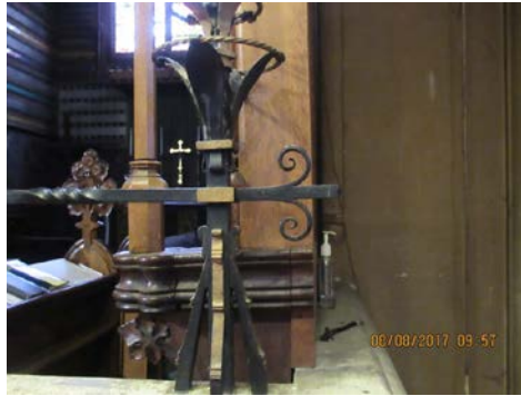
Fig 6 Wrought iron rail – horizontal finial at south end
