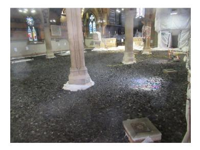
After covering with a mesh limecrete was laid to provide a firm bedding for the tiles which were then re-laid, supplemented by new tiles to match the original ones, although inevitably lacking the patina brought about by years of wear. The new tiles were primarily laid in the centre aisle.
