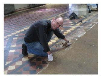
As for the on-site project itself the floor was photographed before the tiles that were left were lifted and removed to Cliveden's workshop for cleaning. Early on asbestos was discovered in the heating tunnel that runs across the front of the church, leading to delay whilst the asbestos was
